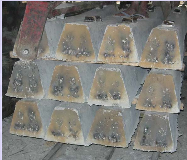
Figure 7-1.1 End of pre-tensioned railway sleepers
